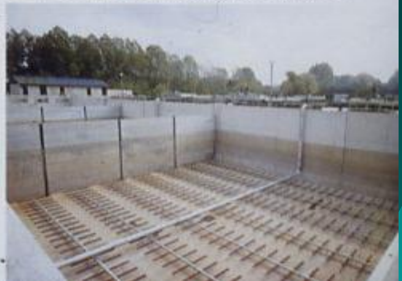
Nürnberg, sewage plant I - 1,2 Mio inhabitants, volume of activated sludge tank = 20.000 m 3
