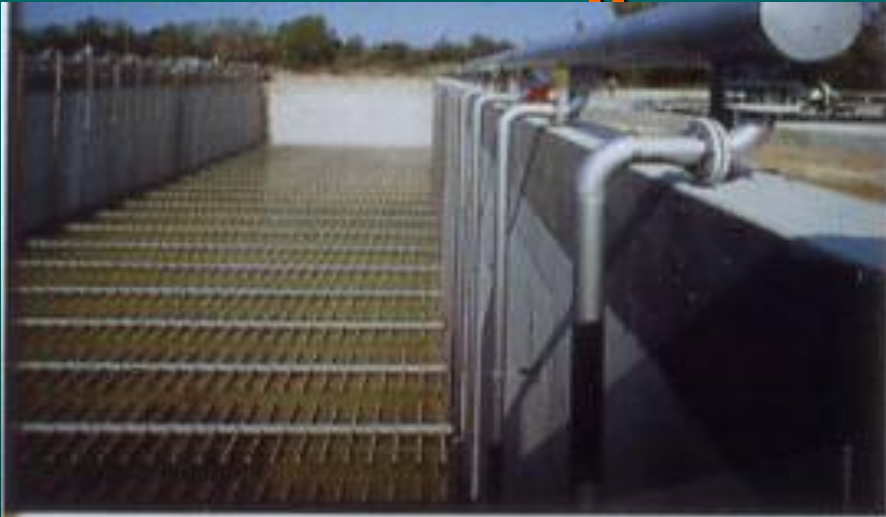
Nürnberg, sewage plant I 1,2 Mio inhabitants, volume of activated sludge tank = 20.000 m 3
