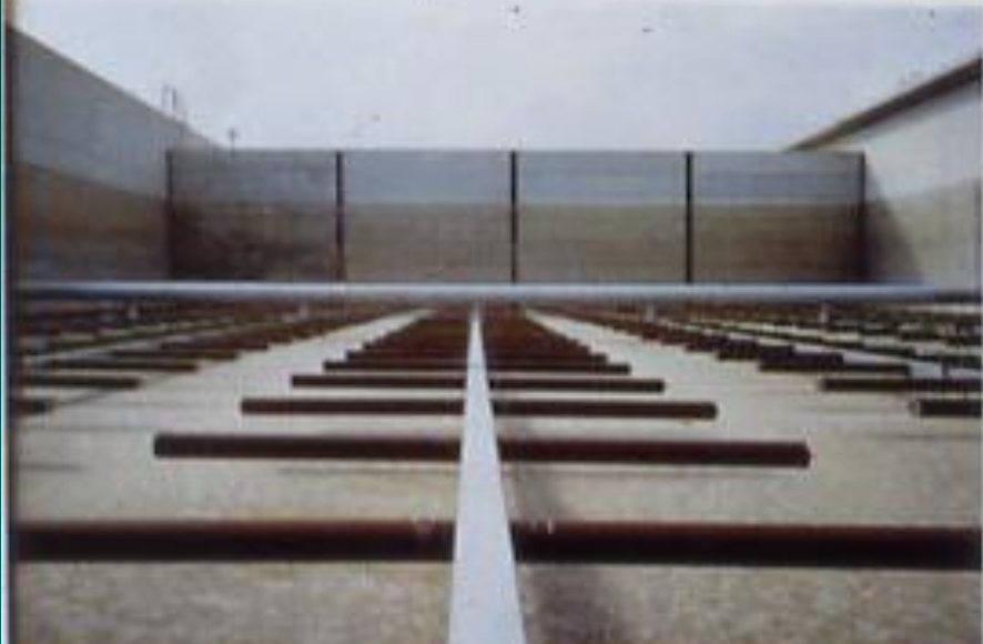
Nürnberg, sewage plant I 1,2 Mio inhabitants, volume of activated sludge tank = 20.000 m 3
