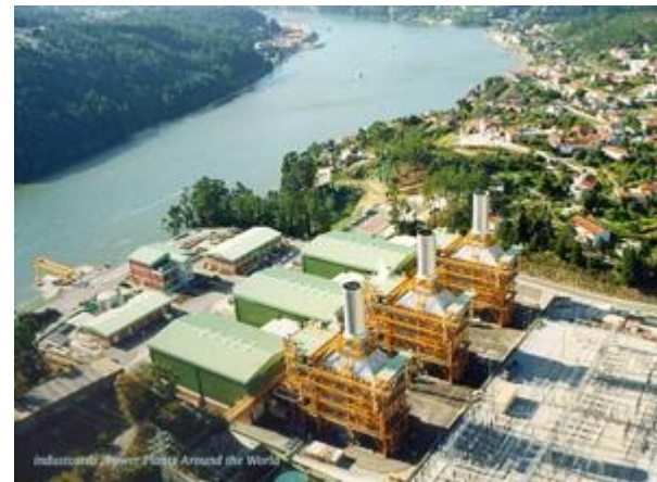
CCTG Power Plant
